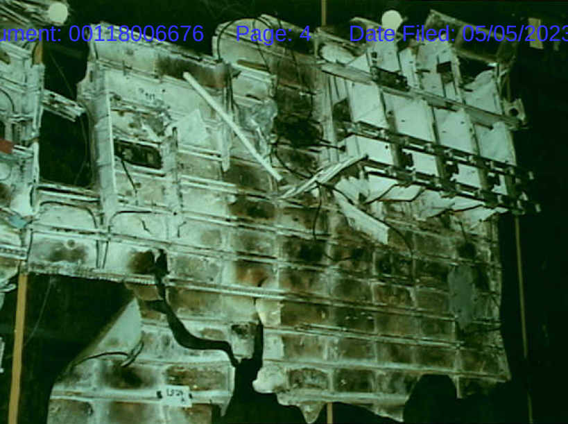
Structures 7 - LF24 - Photo 2
