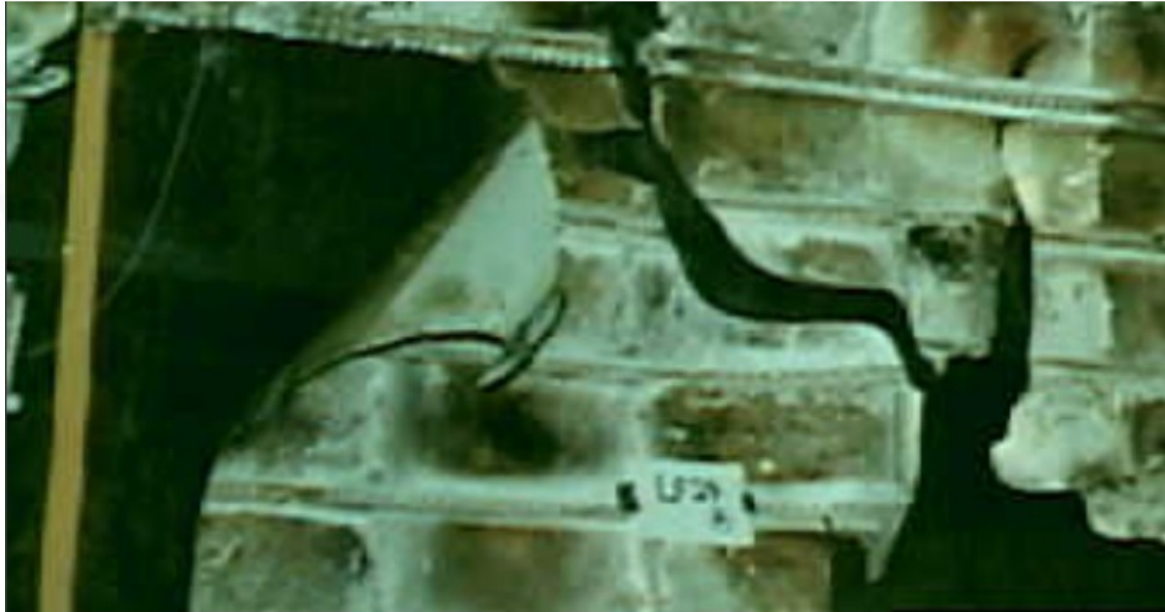
Structures 7 - LF24 - Photo 2
